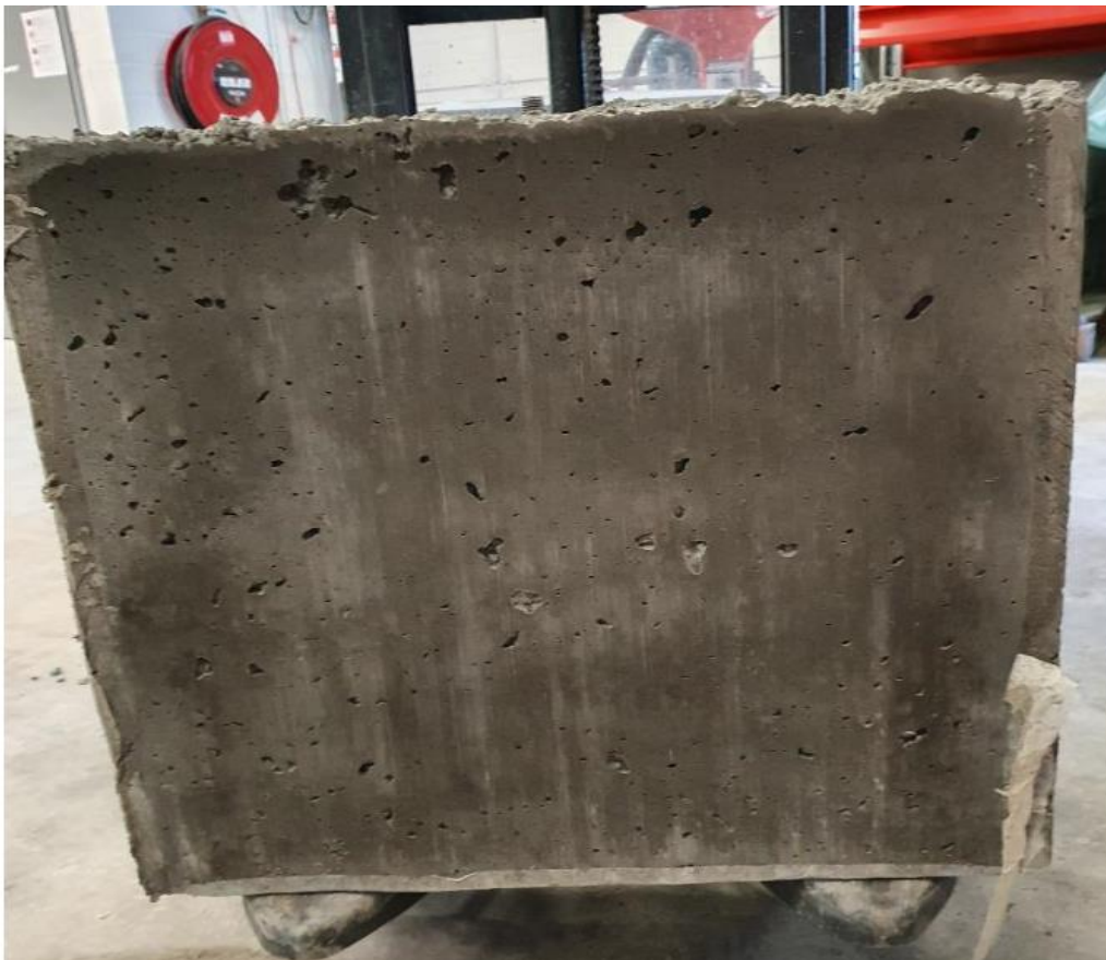
Figure 41 Surface of the concrete
