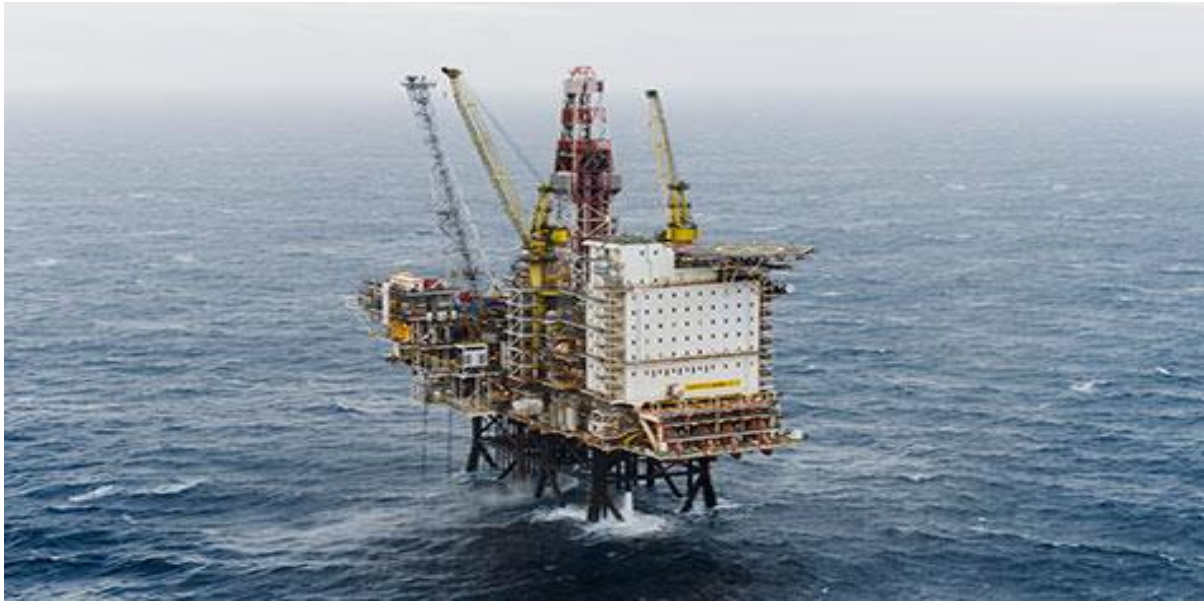
Figure 1: Gyda Platform (Repsol)
