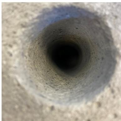
(a) Hole drilled to 243 mm.
