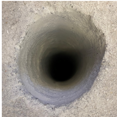
(a) Hole drilled to 400 mm.
