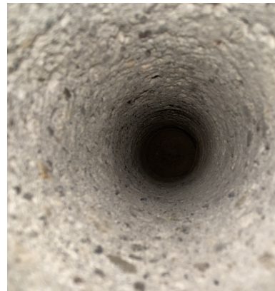
(b) Zoom in off the wellbore to inspect hole quality.
