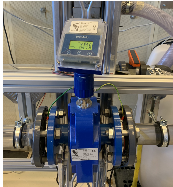
Figure 3.4.: Techfluid XT5 electromagnetic flow sensor
