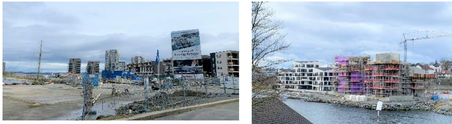
Figure 14: Southeast of Storhaug. Currently under construction.
