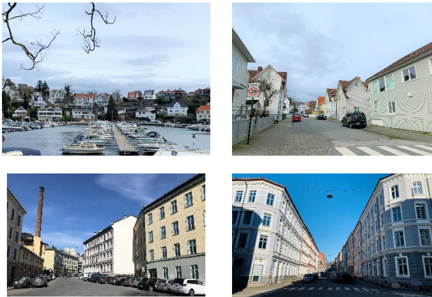
Figure 16: Residence typologies in Storhaug (two upper pictures) and Grünerløkka (two bottom pictures).
