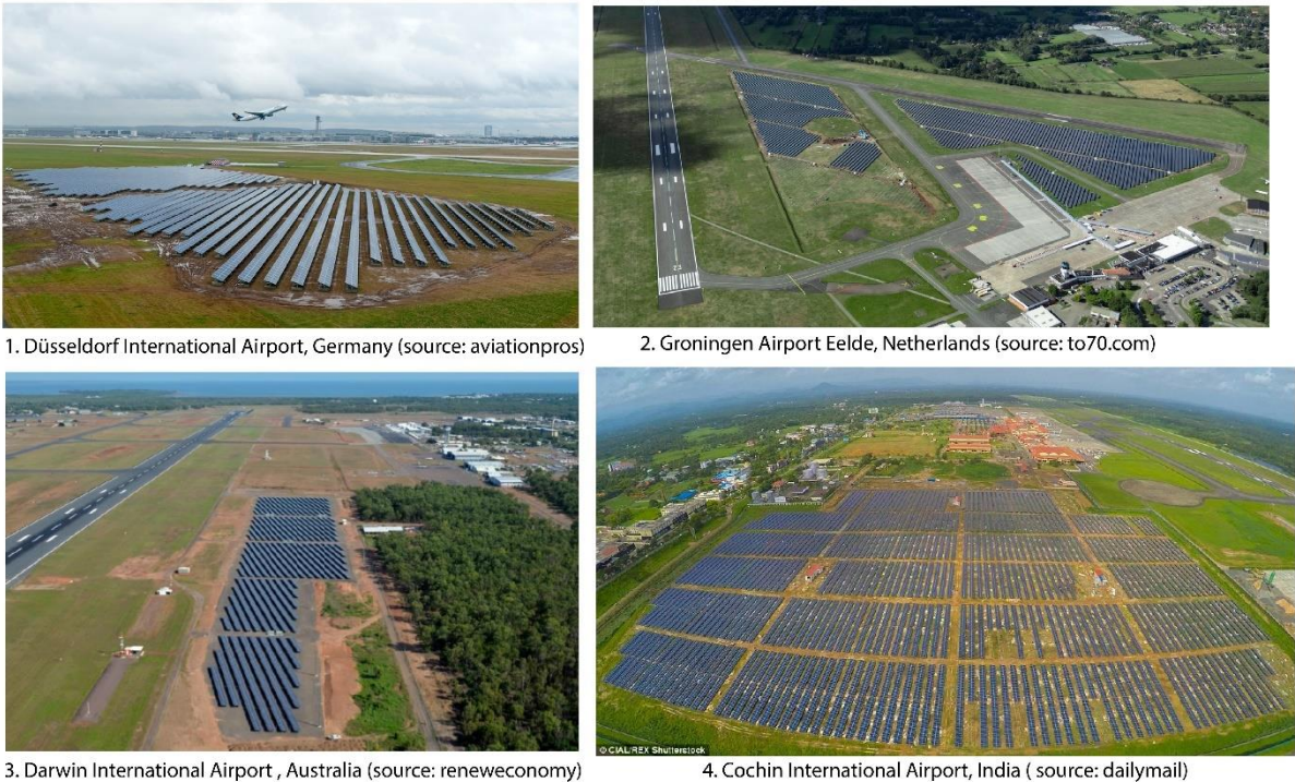
Figure 8: Examples of Large-scale solar PV installations at the Airport
