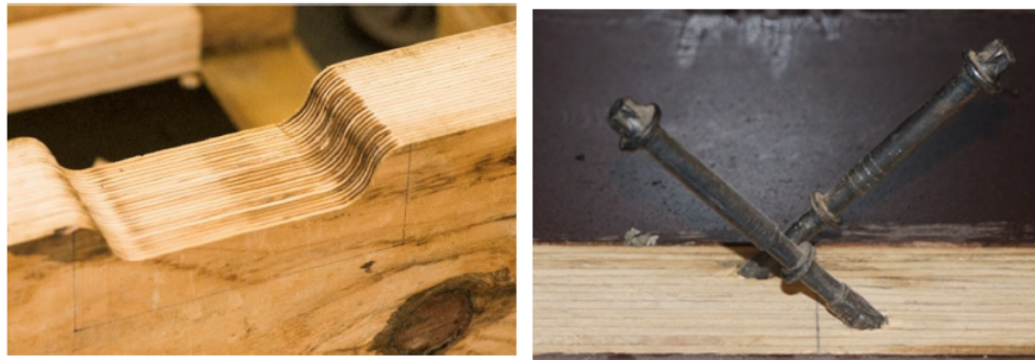
(a) Notche cut in timber.
