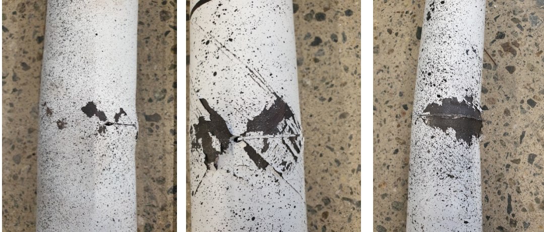
Figure 37: Deformed shape of cracked area (small, medium and large crack respectively)
