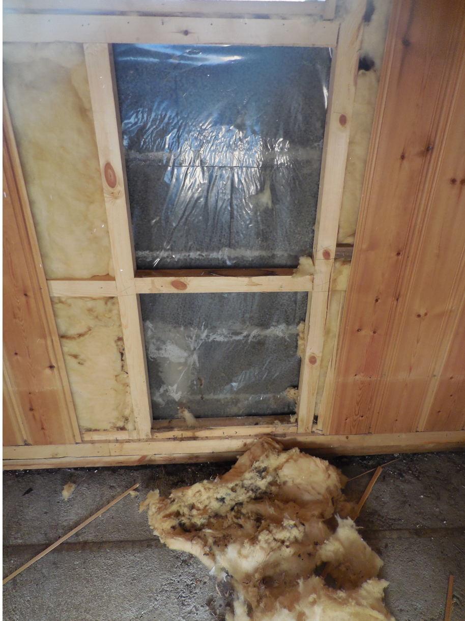
Figure 14: The wall consists of wooden panel, 2×2 studs and sills, 50mm mineral wool insulation, and a vapor barrier installed directly on concrete blocks.
