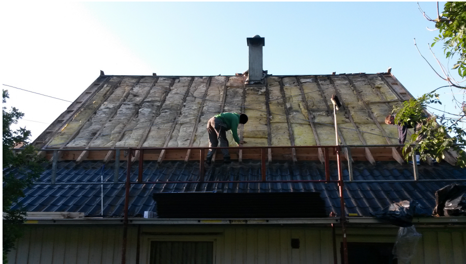
Figure 20: Overview of roof after opening the construction.
