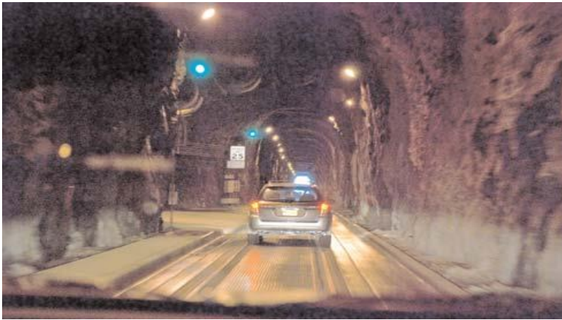
Figure 2.3: Hochtief/ Veidekke JV Tunnel interior: combined-use for road and railway.
