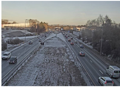
(a) Auglend North
