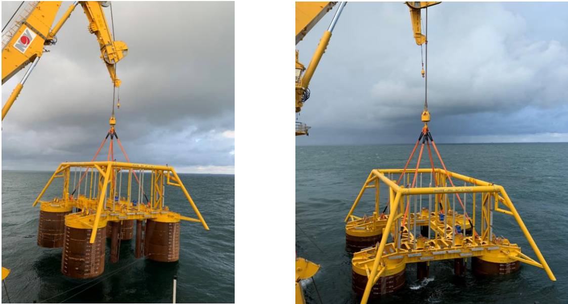
Figure 1-2: ITS deployment at Snorre field [Source: DeepOcean]
