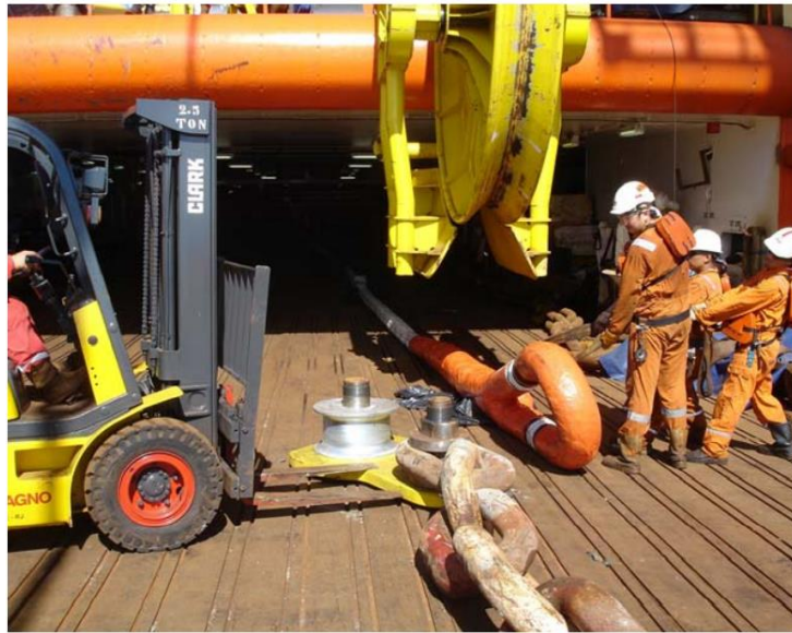
Figure 3.14: Connecting polyester with the H-link to bottom chain [2]
