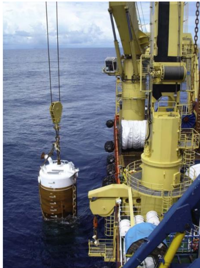
Figure 3.9. Suction pile installation [2]
