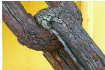
Figure 5.5. corrosion chain above water line [24]
