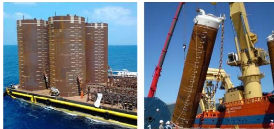
Figure 2.8. Construction of suction piles [8]
