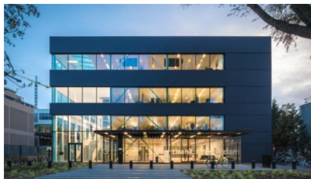
Figure 53 Temporary courthouse in Amsterdam extracted from ( CFP Green Buildings, 2021 )
