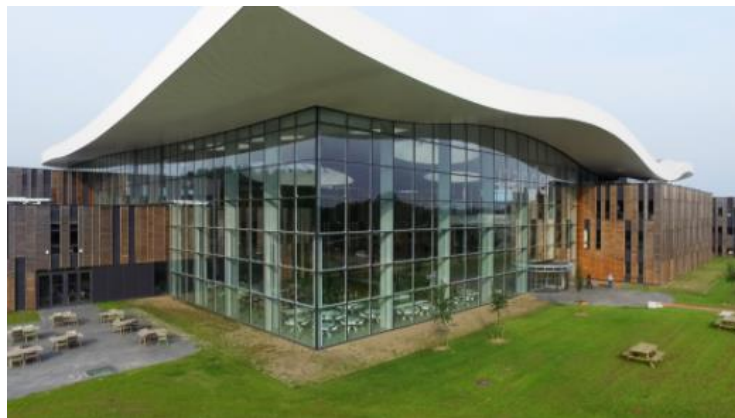
Figure 54 Alliander main office in Duiven extracted from ( CFP Green Buildings, 2021 )
