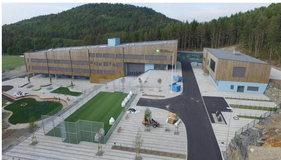
Figure 16 Picture of the building extracted from ( Bogafjell Ungdomsskole, 2021 )
