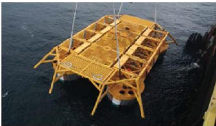
Figure 2–6 Integrated template structure with eight well slots [20]
