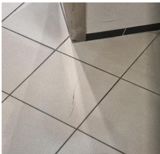
*Figure 2-22 Picture from a local shopping mall, where cracking in tiles could be due to structural movement.*
