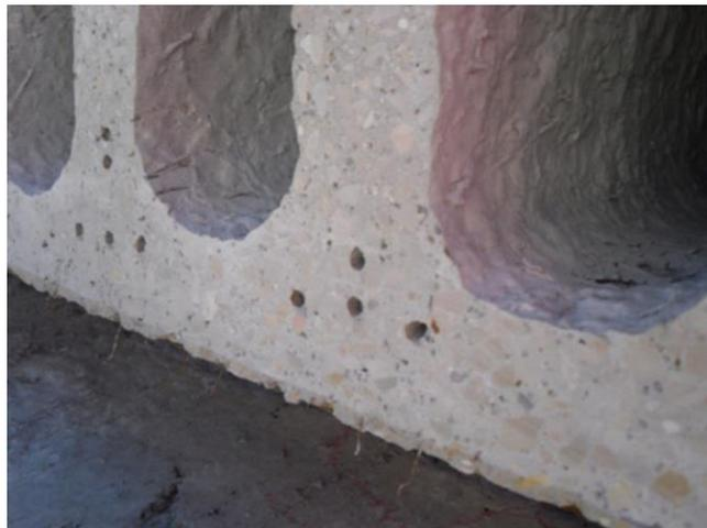
*Figure 2-19 Steel fibers in hollow core slab [20].*
