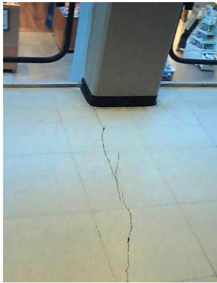
*Figure 2-21 Cracking in tiles [23]*
