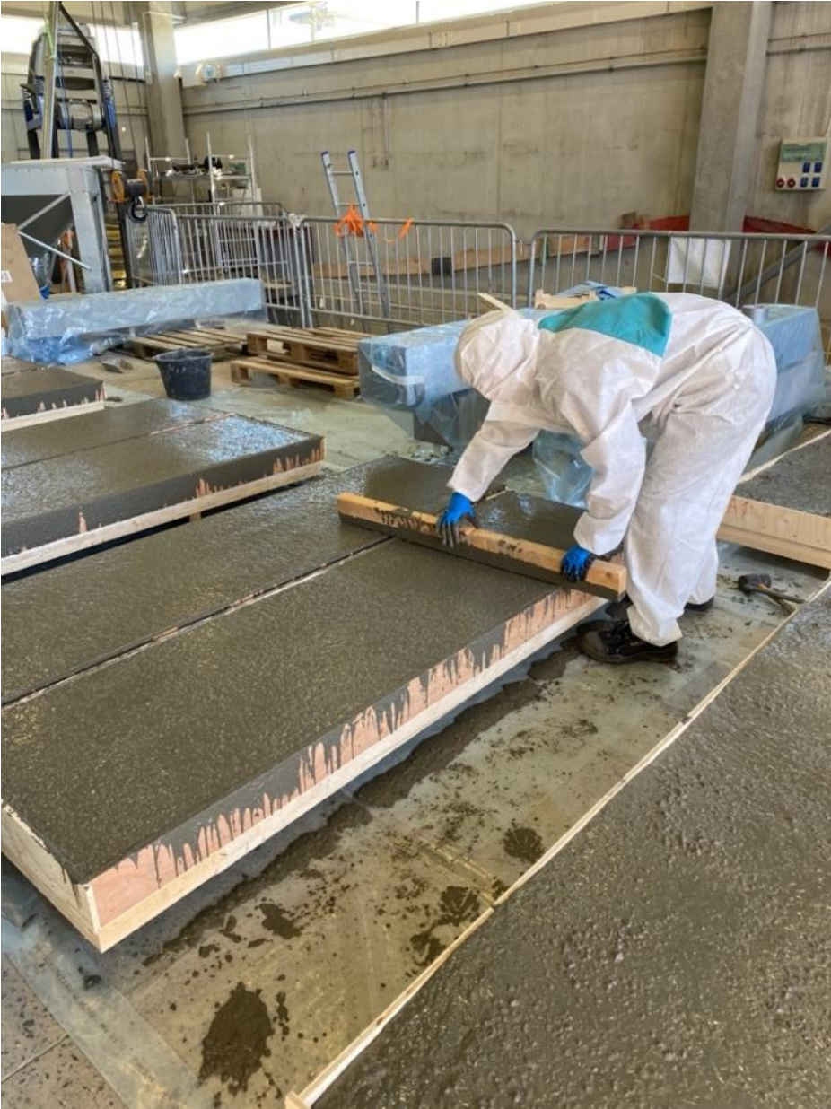
Figure 5-17 Making the concrete smooth and levelled
