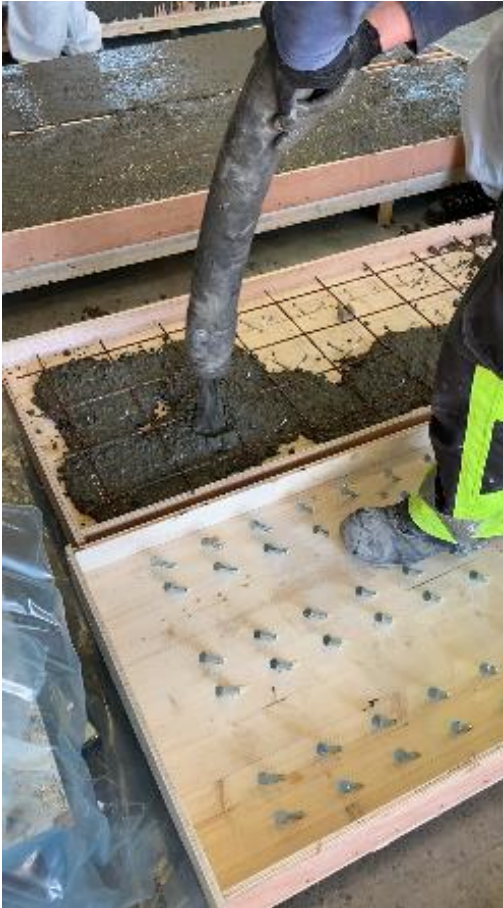
Figure 5-15 Pouring concrete onto the CLT slabs, both types are shown
