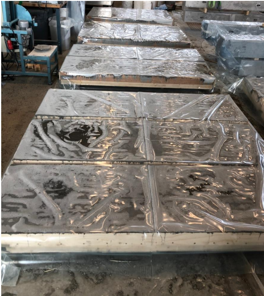
Figure 5-19 Plastic covering the CLT-concrete composite slabs for curing
