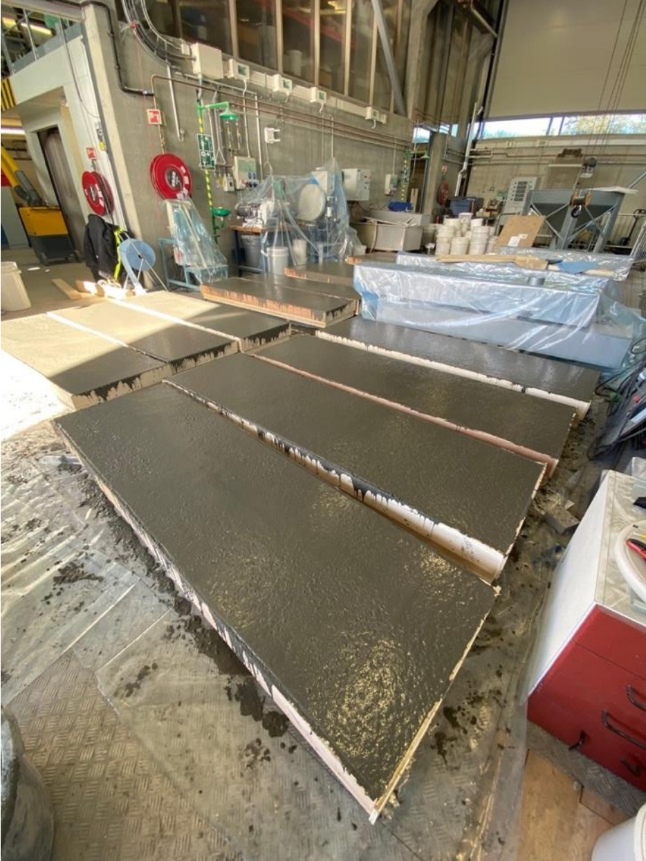
Figure 5-18 Finished casted concrete
