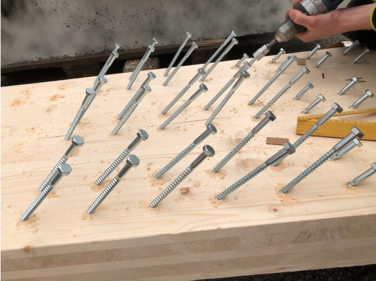
Figure 5-10 Fastening the KOP screws into the CLT slab
