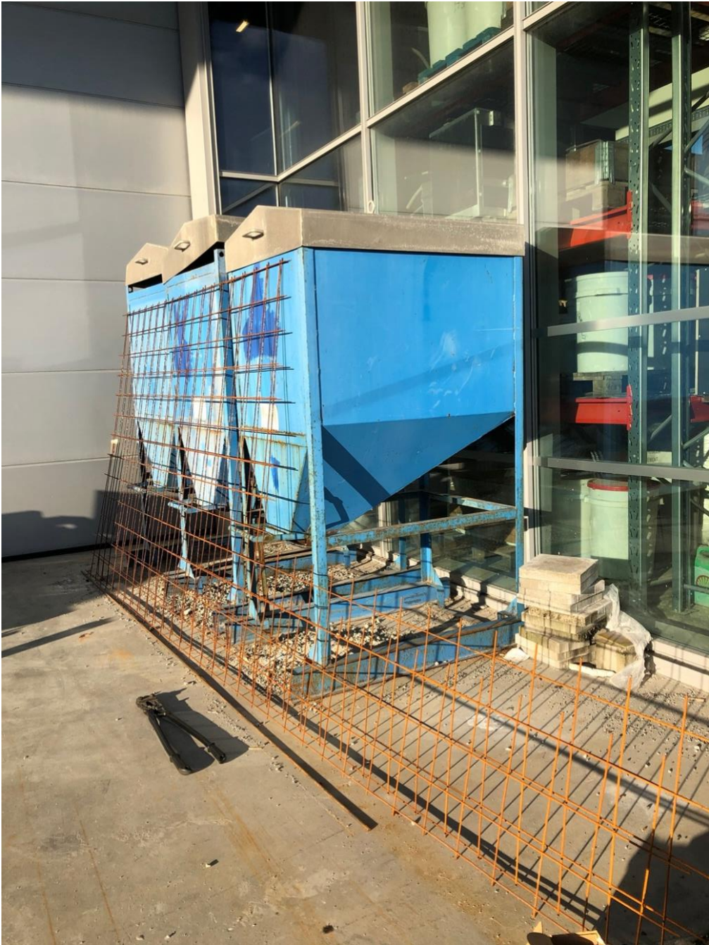
Figure 5-5 Bolt cutter and the steel reinforcement mesh
