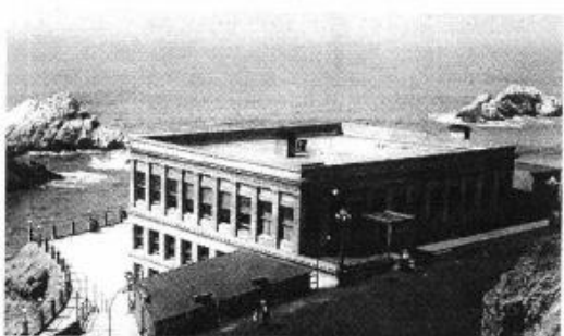
1910 - After a fire in 1907 the Cliff House was reconstructed of fireproof concrete and steel.
