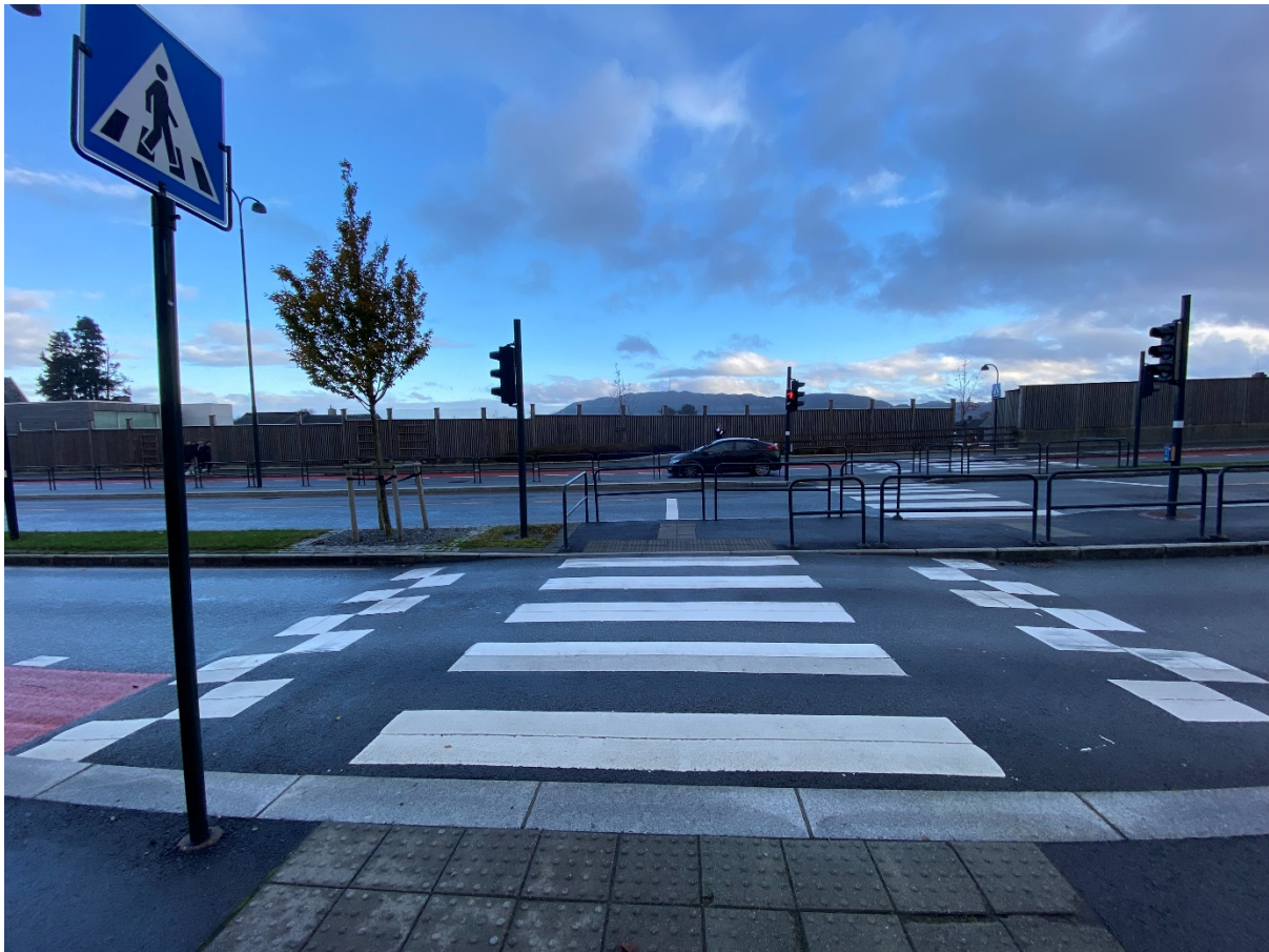
Picture 6: Zebra-crossing near the Lyngnesveien bus stop. Photo by Vieira (2021).
