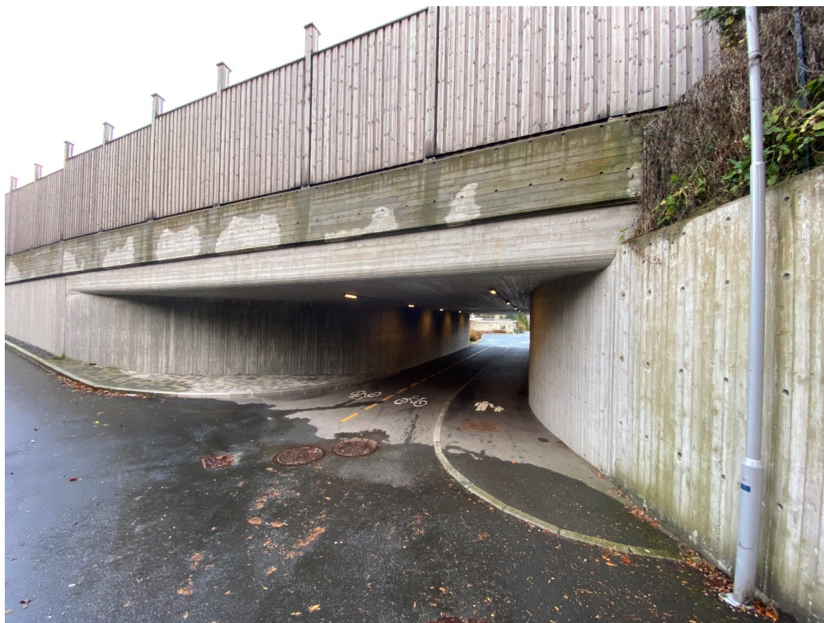
Picture 4: Internal aspect of Lyngnesveien underpass. Photo by Vieira (2021c).
