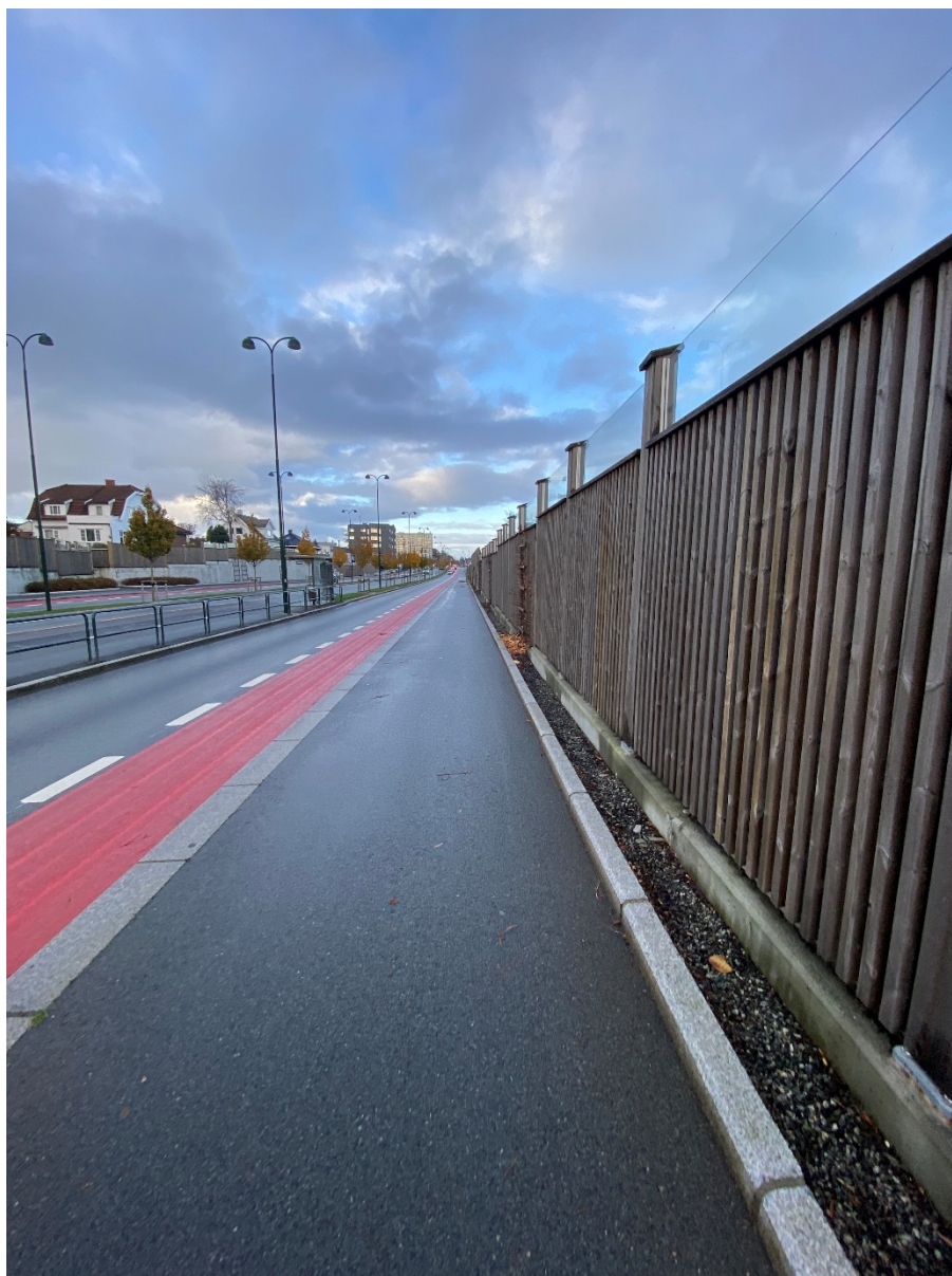
Picture 9: Noise abatements near Lyngnesveien bus stop. Vieira (2021c)
