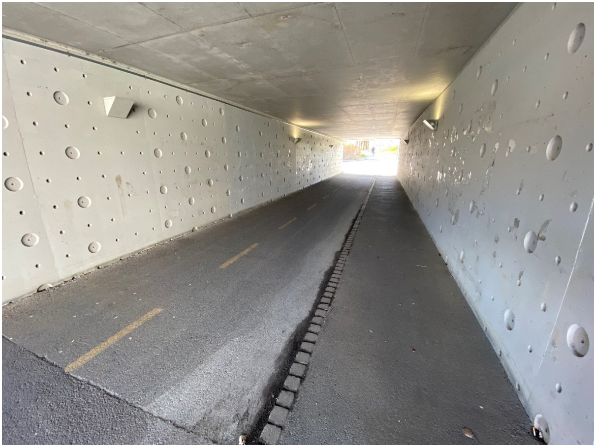
Picture 2: Interior of Eikeberg underpass. Photo by Vieira (2021c).
