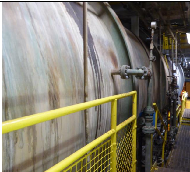
Picture 11. Vessel not insulated, picture taken from south side.
