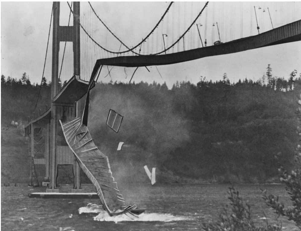
Figure 0.1 Collapse of the Tacoma Narrows Bridge at 11:15 AM on 7 November 1940 (Scott, 2001)
