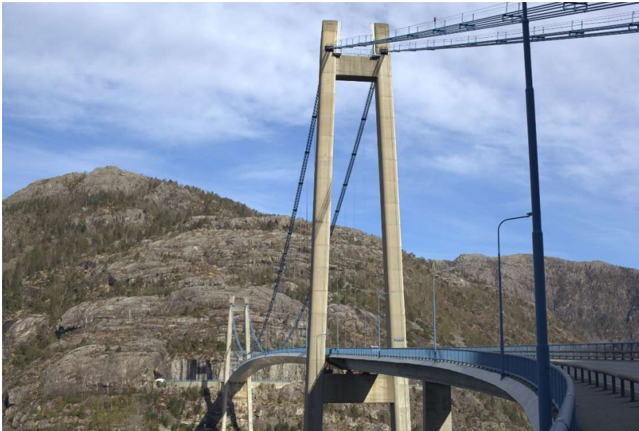
Figure 1.1 Picture of the Lysefjord suspension bridge. Photo: Fredrik M. Pedersen
