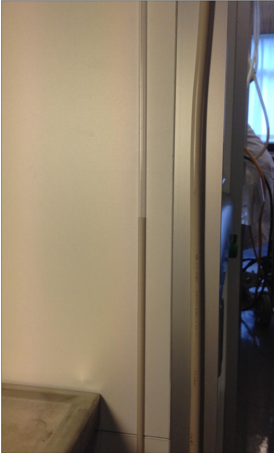
Picture 9: Picture taken after the light fluid has been inserted into the pipe. [P1]
