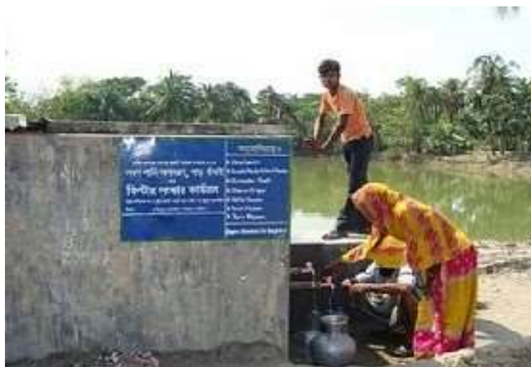
Figure 43 – Pond-sand filter system
