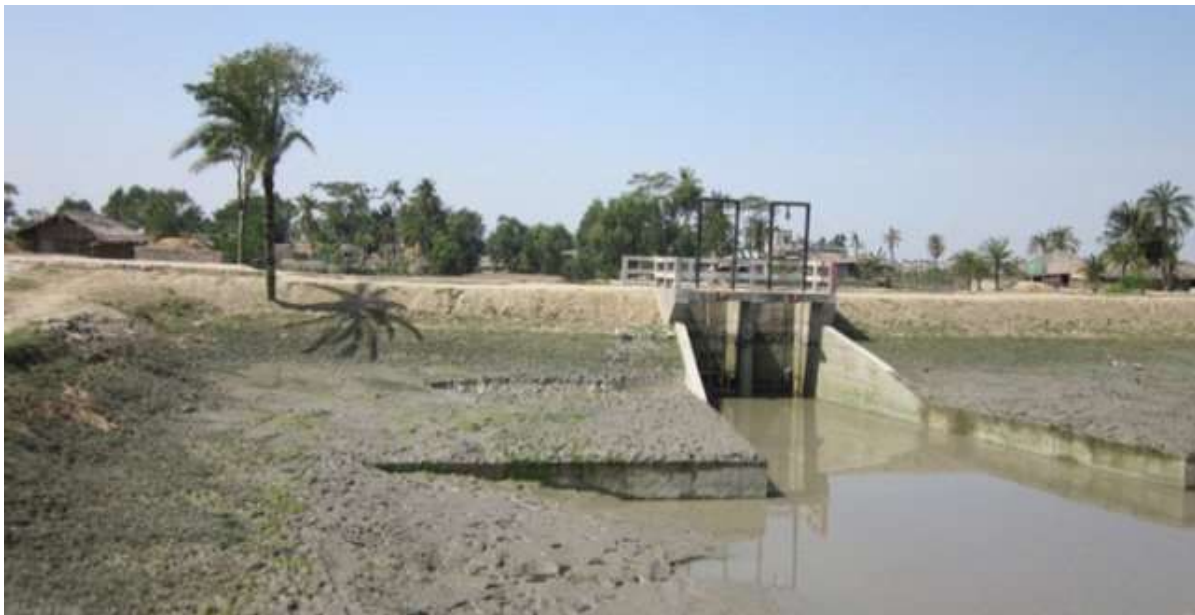
Figure 50 - Polder with earth embankment and gate structure
