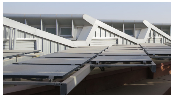
Figure 4.31: Dirt and sand on the solar panels on top of the residential buildings (I. Moxnes)
