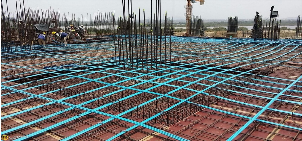
Figure 9 – Example of post-tension cables on a construction project (Daily Engineering, 2021)
