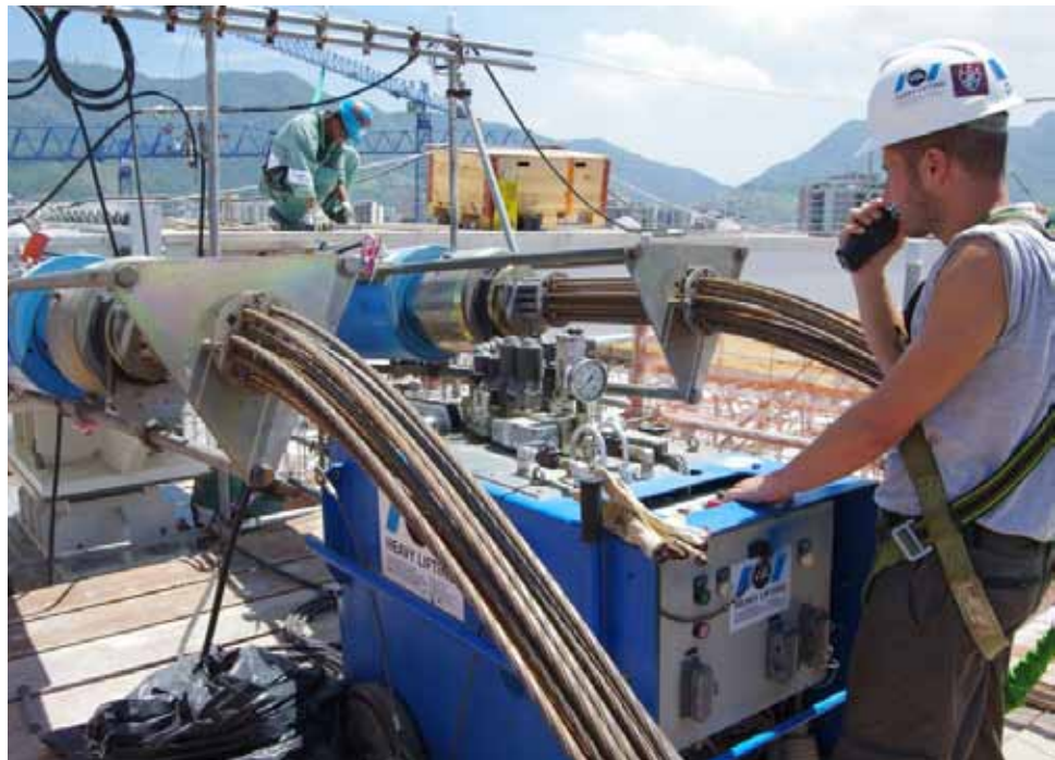
To lift the cable-net roof of a major stadium, two strand jacking units were installed at each lifting point on the compression ring. Each pump served up to seven lifting points. Maracanã Stadium, Rio de Janeiro - Brazil (2013)
