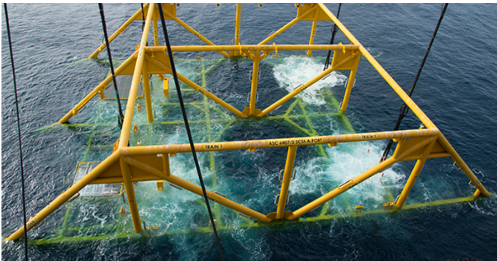
Figure 1 - 2 Splash zone crossing of a subsea template [7].
