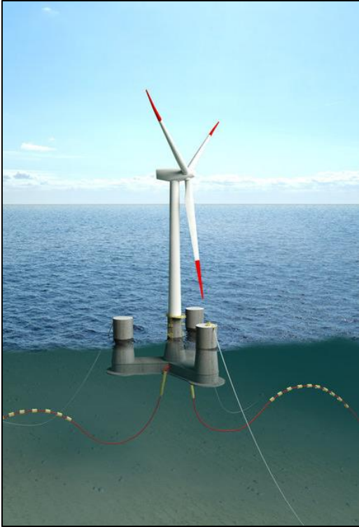
Figure 20 The LIFES50+ OO-Star Wind Floater Semi 10MW structure 10-MW OO-Star floating wind turbine (Yu, 2017)
