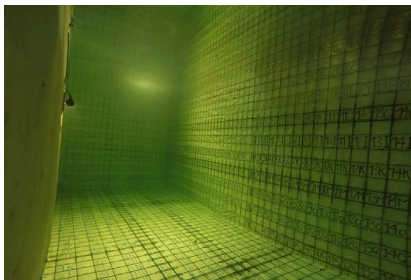
Figur 6 Pool after completion
