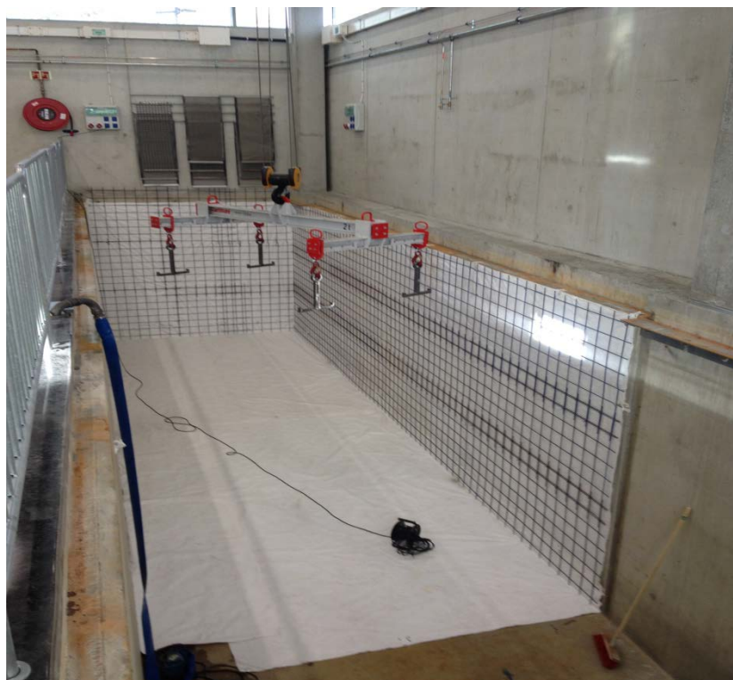
Figur 5 Pool under construction
