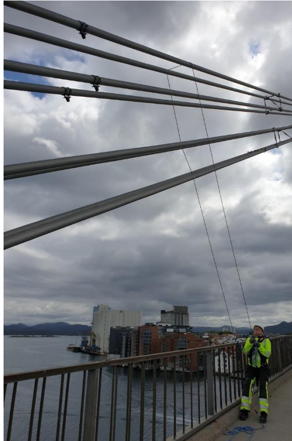
Figure 43 Manually pulling the cable. Photo by Jasna B. Jakobsen, UiS
