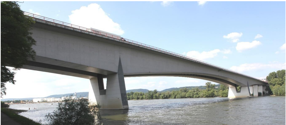
Figure 3 Bendorf bridge, visited by the municipal delegation [4]
