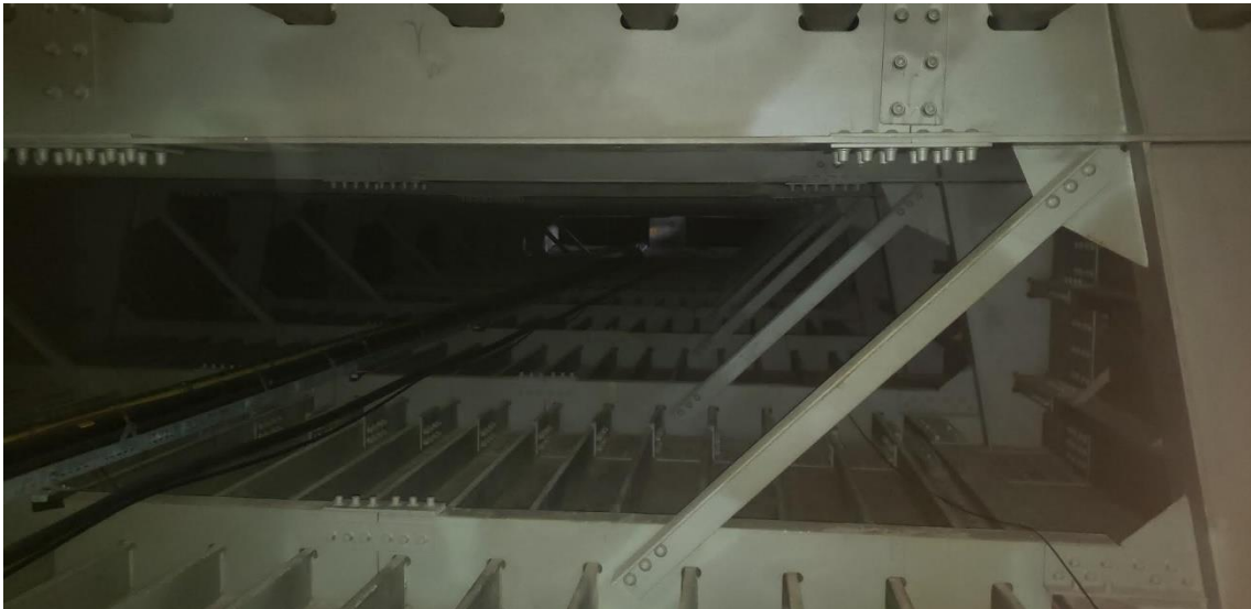
Figure 27 Steel box girder at the main span
