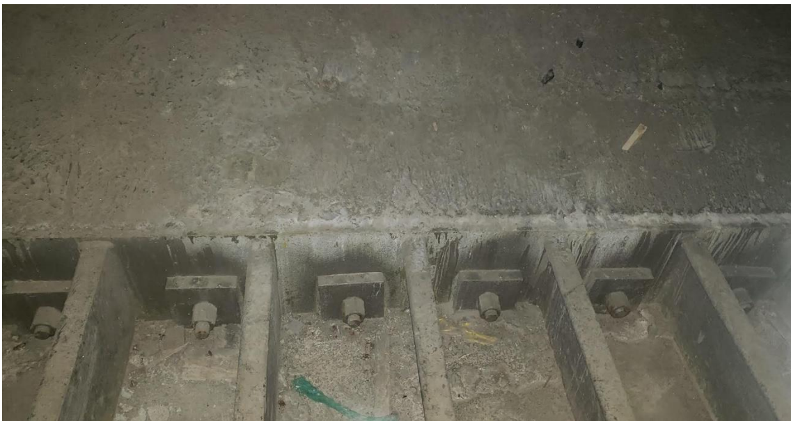
Figure 28 Connection between concrete girder (top) and steel girder (bottom)
