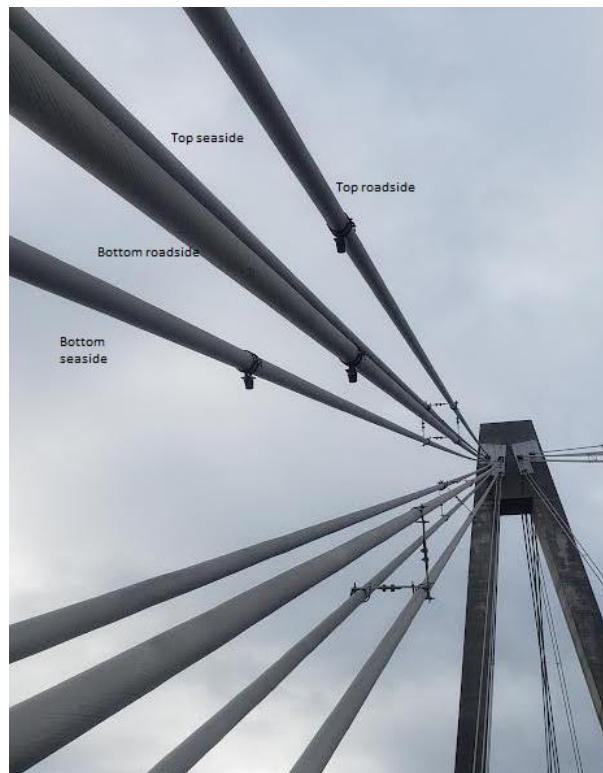
Figure 31 Sensors on the cable bundle after 20/04/2021
