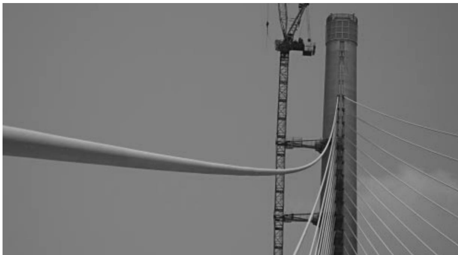
Figure 42 Visible sag on Stonecutters Bridge [1]
