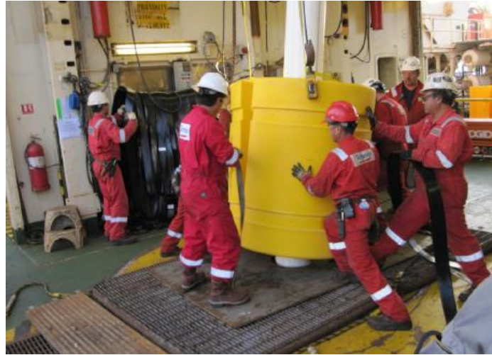
Figure 8-8 the Installation of buoyancy Module onto the Riser (Beattie et al., 2013)
