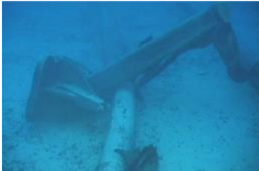
Figure 3-2 - Third pipeline (20 inches) laterally displaced 43 meter with anchor under (Orsolato, et al., 2011)
