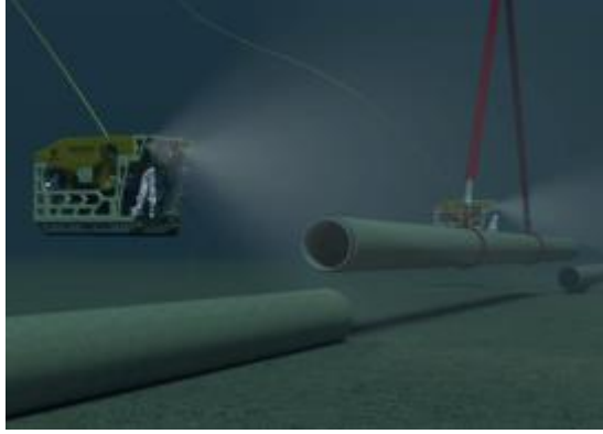
Figure 2-20 - Lowering pipe segment between two plugged pipe ends (Berge, et al., 2015)
