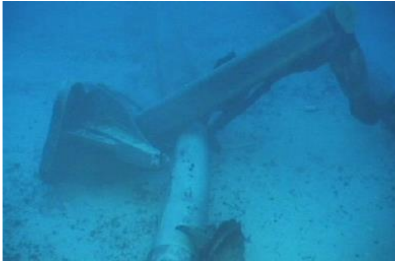
Figure 2-7 - Anchor stuck under a pipeline, leaving the pipeline damaged and lateral displaced by bending (Orsolato, et al., 2011)
