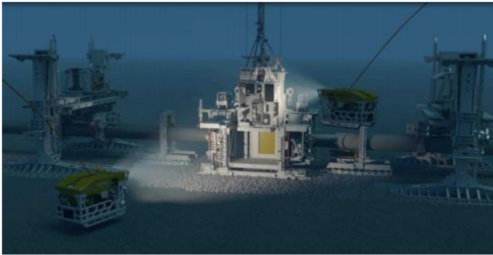
Figure 2-21 - Remote welding system mounted on a pipeline joint
