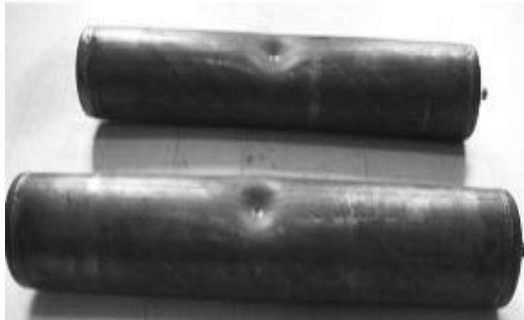
Figure 2-3 - Dent on pipeline (Allouti, et al., 2014)
