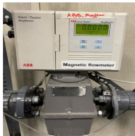
Figure 4.3: Magnetic Flow Meter
