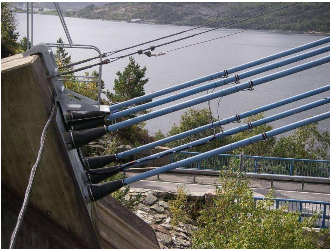
Figure 4. Position of sensor along each main cable at each anchor [26]
