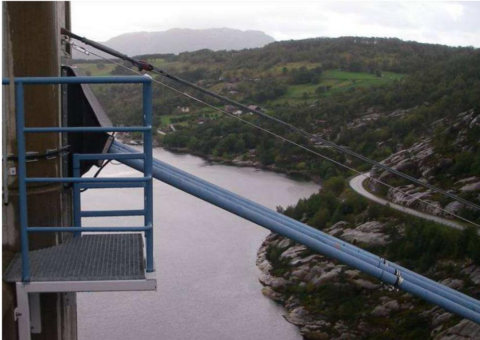
Figure 5. Position of sensor along each main cable on the backstay side of each pylon [26]
