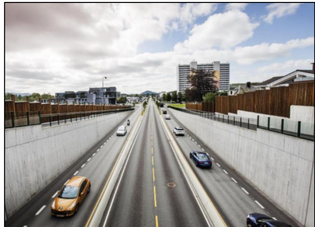
Figure 28: Photo of the busway at Hillevåg (Tønnessen, 2020).
