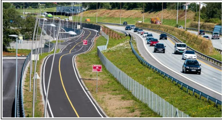
Figure 29: A completed section of the cycle highway between Stavanger and Sandnes (Refvem, 2020).
