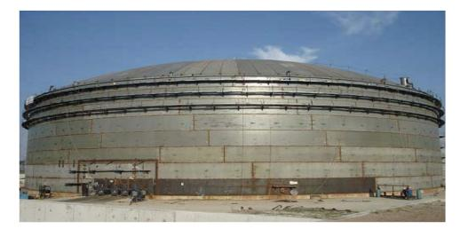
Figure 5.3: Internal floating roof tank
