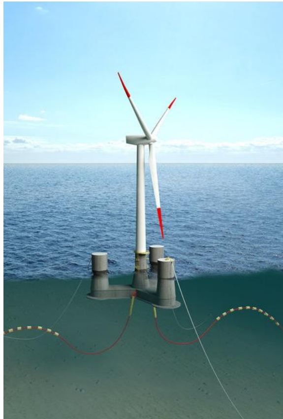
107 Figure 1 The 10-MW OO-Star floating wind turbine [13].
