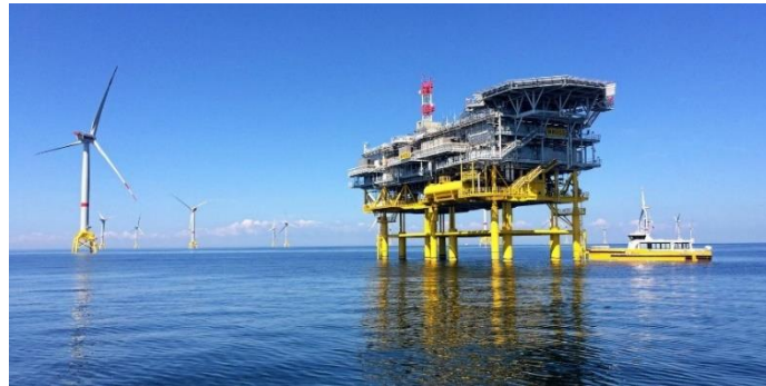
Figure 8: Offshore wind park and substation [55].
