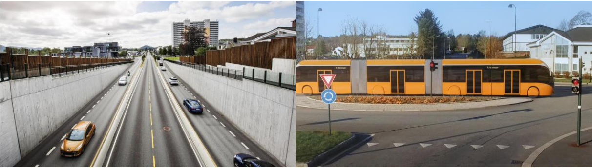
Figure 2.8 The buses have dedicated lanes and drive straight through right-of-way roundabouts (Rogaland fylkeskommune, 2020a)
