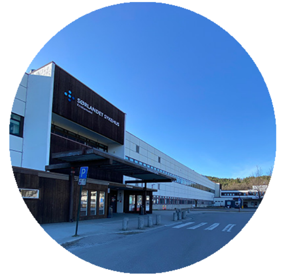
Figure 58: The main building and the hospital entrance
