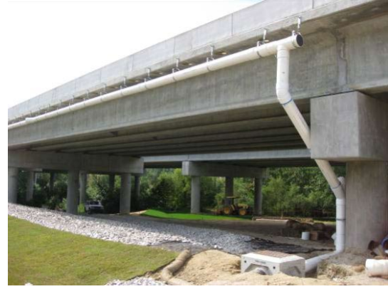
Figure 10 Water delivery system for bioretention and bioswale (World Environmental and Water Resources Congress. (2010))
