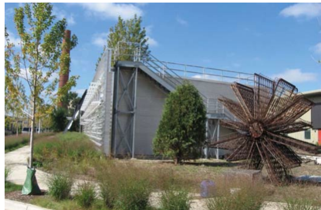
Figure 7 Building in Chicago features a green roof, permeable paver and bioswales ( EPA Office of Wetlands, Oceans and Watersheds. (2010))
