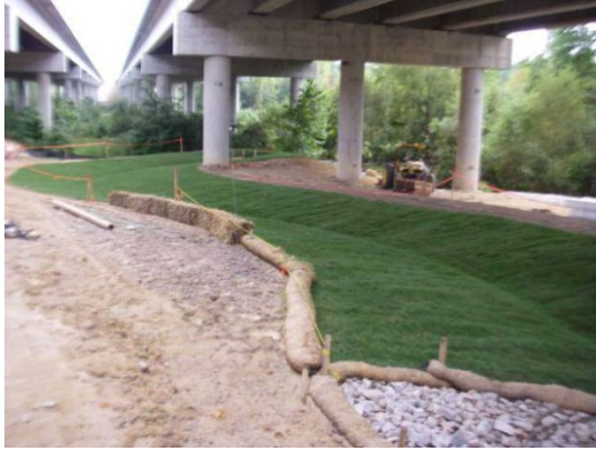
Figure 9 Bioswale at Mango Creek (World Environmental and Water Resources Congress. (2010))
