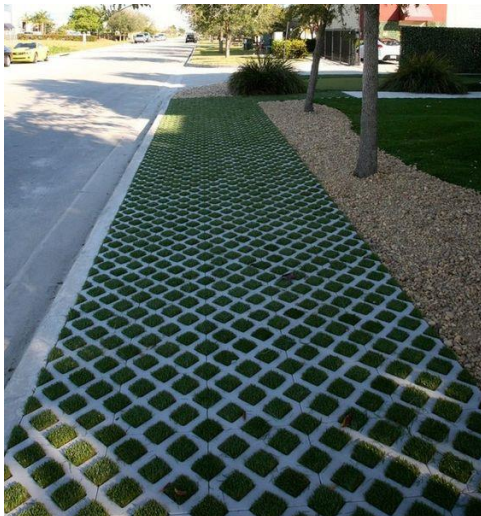
Figure 8.25. Example of permeable pavement for parking
