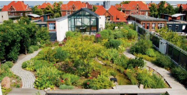
Figure 5.14. Intensive green roof
