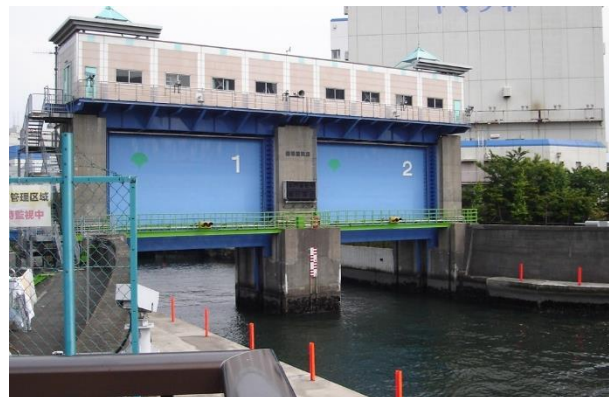
Figure 5.21. Sluice gate. Tokyo, Japan
