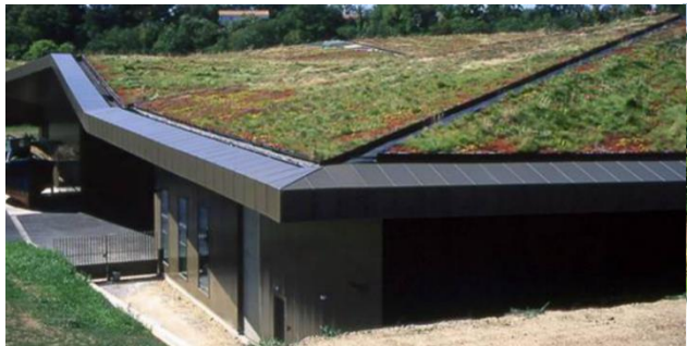
Figure 5.13. Extensive green roof
