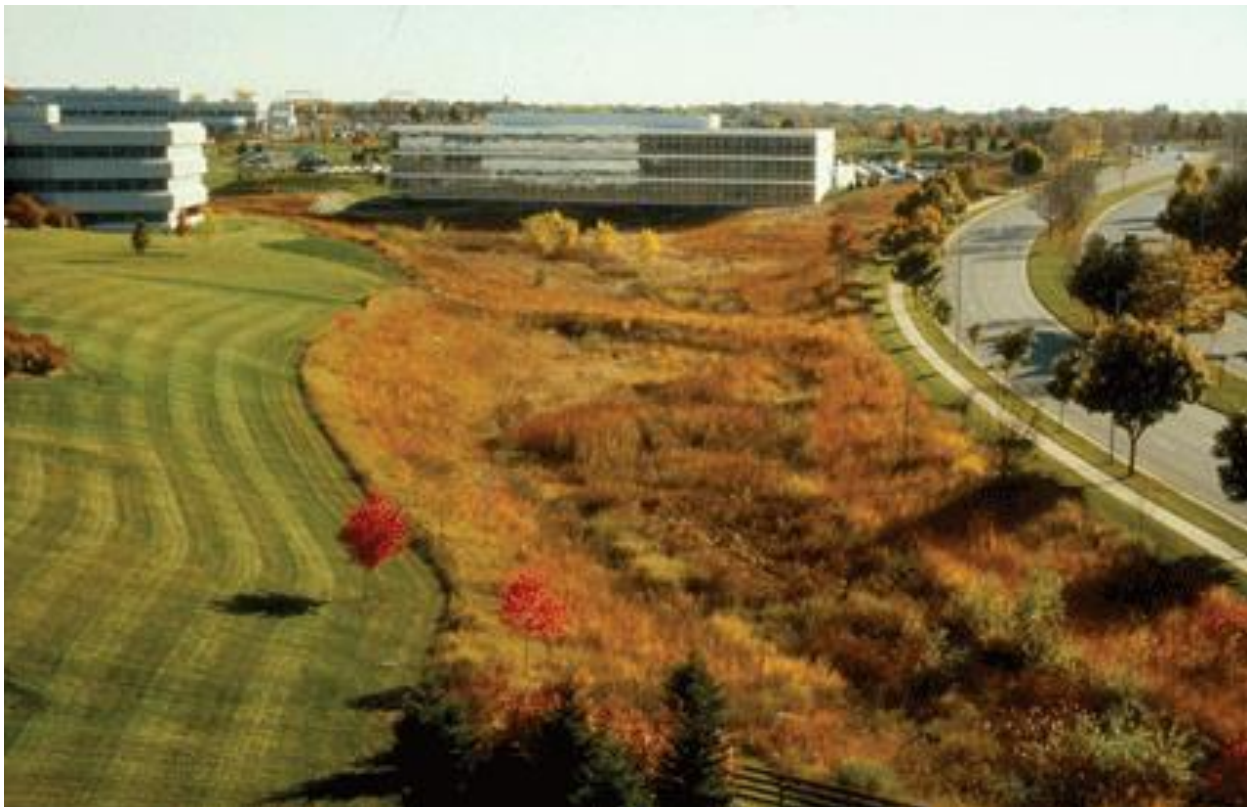
Figure 5.31. Larger bioswale (NRCS, 2005)
