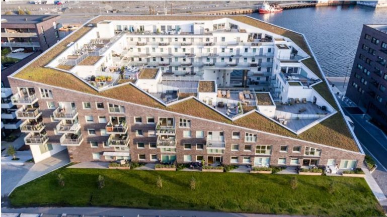
Figure 8.6. Example of extensive green rooftops. Sjørenga blokk 6 by Mad arkitekter
