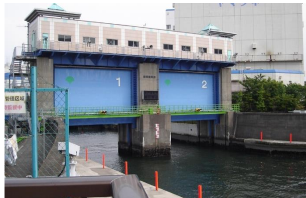
Figure 5.21. Sluice gate. Tokyo, Japan
