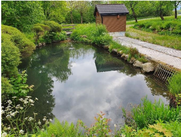
Figure 5.40. First pond in a wetland system near Mosvatnet, Stavanger. Used to treat stormwater before it reaches the lake.
