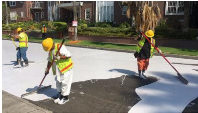
Figure 5.54. Workers painting the pavement white to combat high temperatures.
