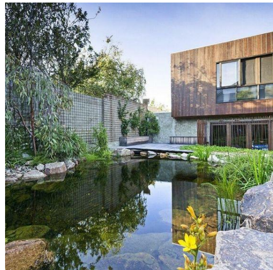
Figure 8.17. Example of urban pond closely connected to buildings
