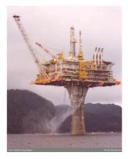
**Figure 1.** The Draugen platform ready to be towed to site in 1993. Note the slender concrete shaft and the widening at the top to support the topside facilities.
