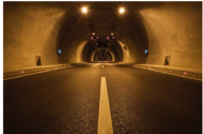
Figure 5. Double-lane one-way road tunnel.
