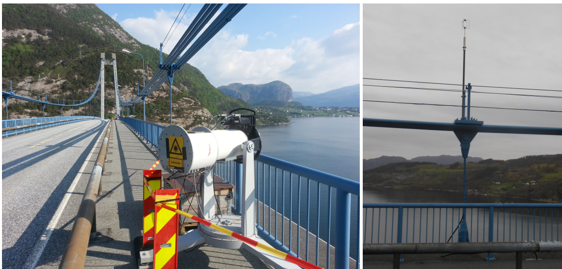
Figure 2. Wind sensors on the Lysefjord Bridge: (left) Short-range WindScanner [5] and (right) WindMaster Pro 3D sonic anemometer at midspan.
