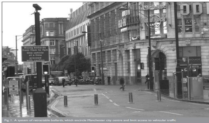
Fig. 1. A system of retractable bollards, which encircle Manchester city centre and limit access to vehicular traffic
