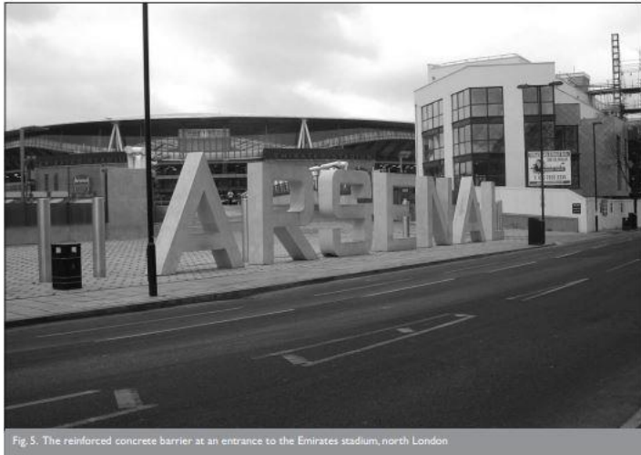
Fig. 5. The reinforced concrete barrier at an entrance to the Emirates stadium, north London
