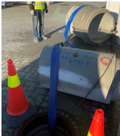
(a) Pump cable positioning to avoid angles for smooth flowthrough
