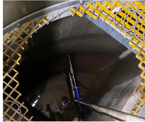
(b) YSI probe lowered toward outlet pipe
