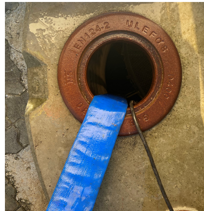
(b) Pump cable into inlet chamber
