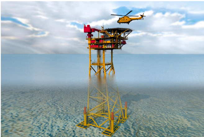
Fig. 5. An example of offshore Jacket platform operating in the Bohai continental shelf.
