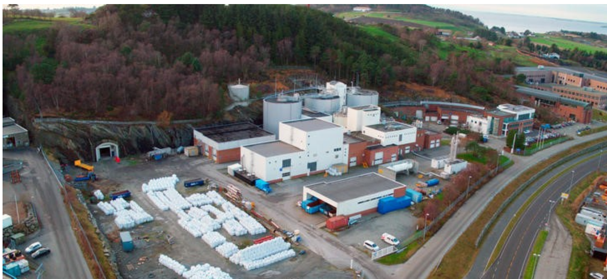
Figure 1.1 IVAR SNJ WWTP (Photo: ivar.no).
