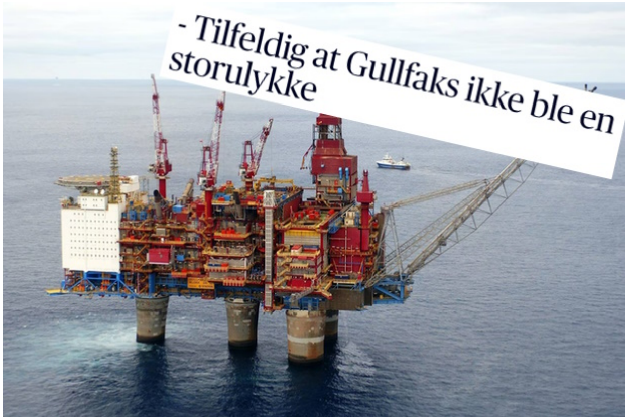
Figure 3.4.1: Picture of the Gullfaks A platform in the North Sea, along with the headline of an article in Aftenposten that implies the possibility of a major incident on the field. Photo: Øyvind Hagen, Statoil
